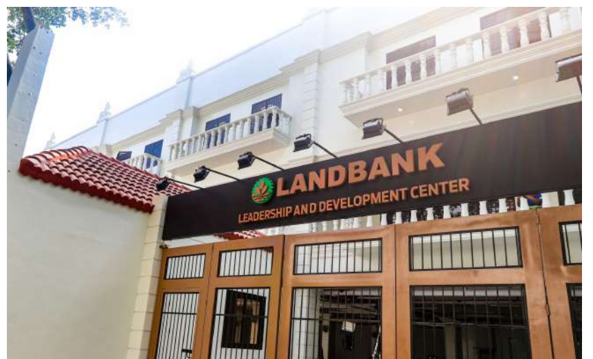
The LANDBANK Leadership and Development Center is located along Cabildo St. in Intramuros, Manila.
